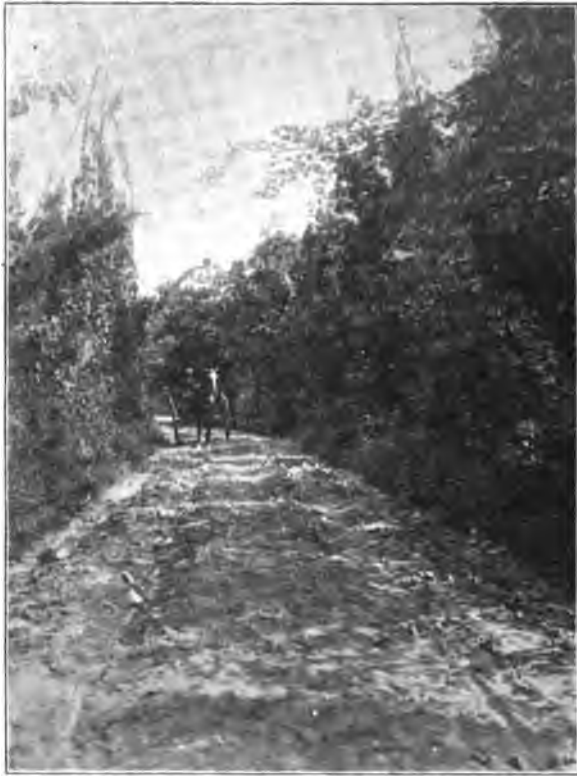
Clove Road, Passaic Co., before improvement.
